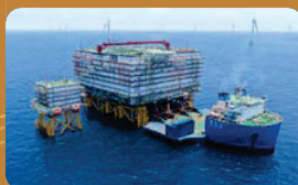
COSCO 25,000-TONNE OFFSHORE PLATFORM INSTALLATION
