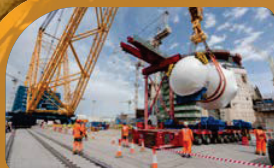
BIG CARL LIFTS HINKLEY POINT C'S SECOND REACTOR
